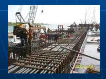
Wharf designs use high strength steel to reduce steel quantity and improve constructability
